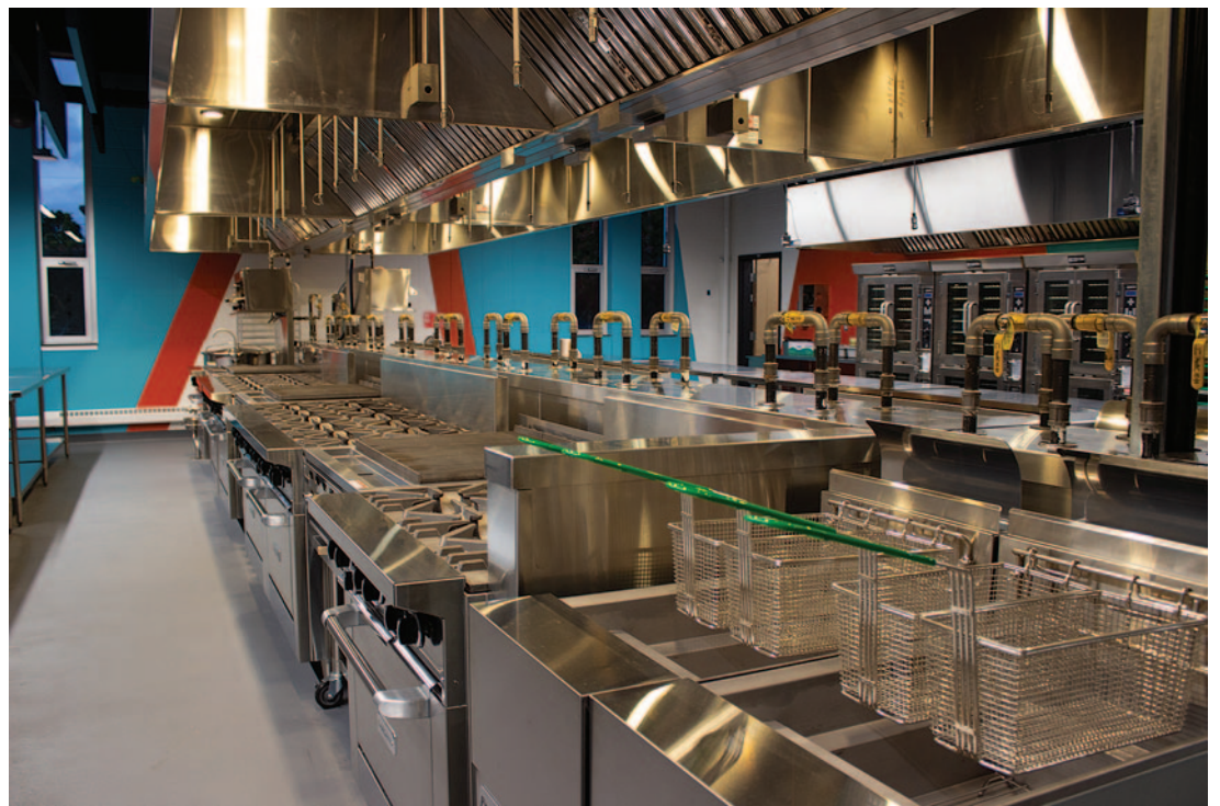
A look at one of the new kitchens.
