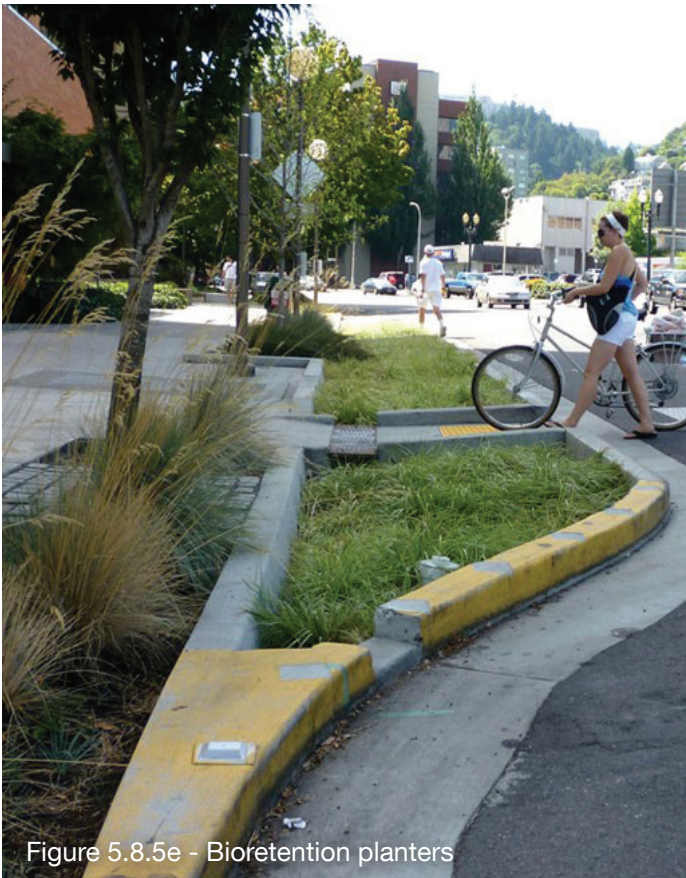
Figure 5.8.5c - Bioretention planters
